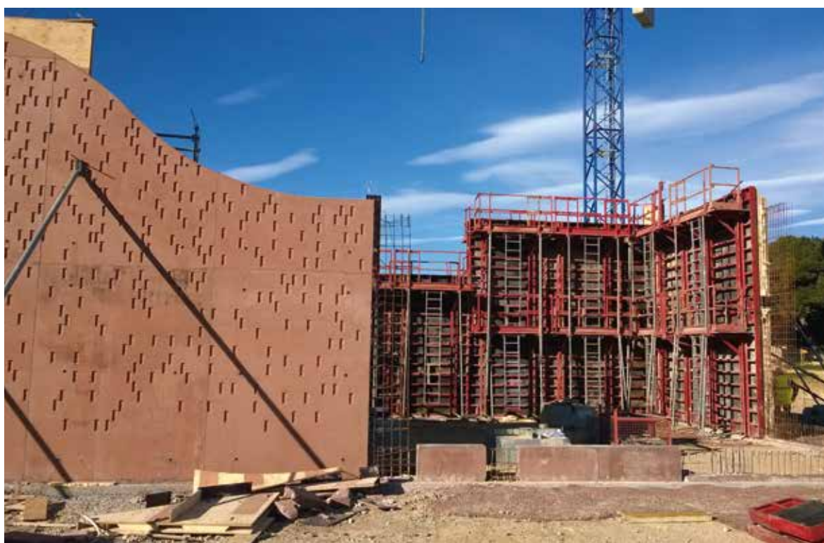
SOGEA / RAZEL BEC – Station de pompage Mejanelle
